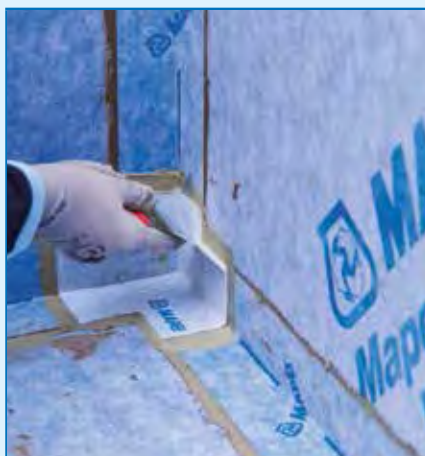
Aplicarea piesei de colt intern MAPEGUARD IC cu MAPEGUARD WP ADHESIVE
