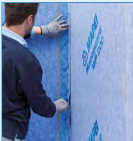
Aplicarea MAPEGUARD ST cu adeziv MAPEGUARD WP ADHESIVE
