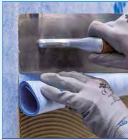
Aplicarea celei de a doua fasii de membrana MAPEGUARD WP 200 (prin alaturare)
