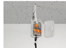
Pendant light connection in a suspended ceiling
