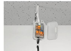
Pendant light connection in a suspended ceiling
