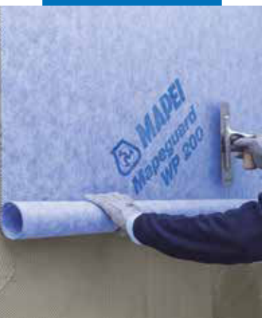
Aplicarea Mapeguard WP 200
